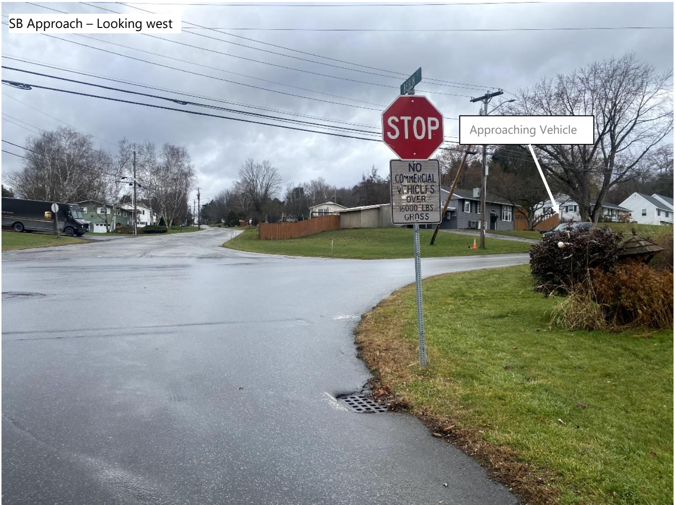
Figure 4 Partial Obstruction at Stop controlled approach
